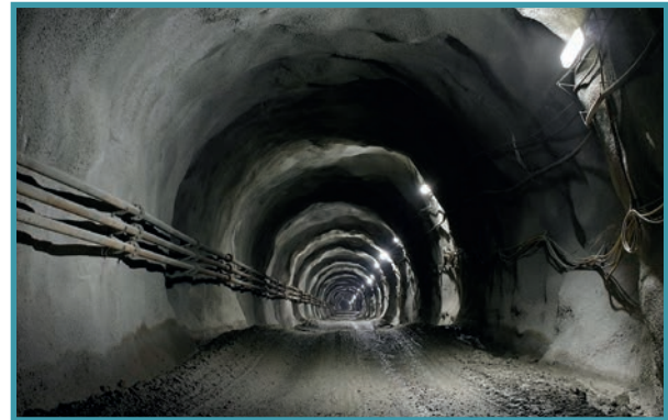
Shotcrete Application in Mines
