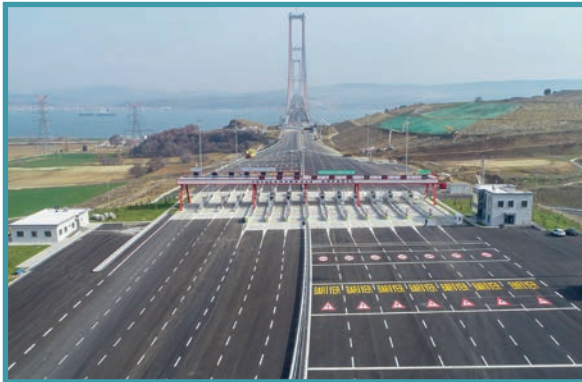
Highway Toll Constructions
